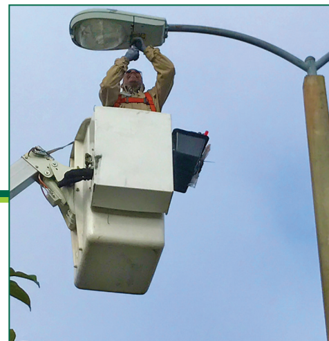
On the Job: Lon Crawford at work repairing a street light.
