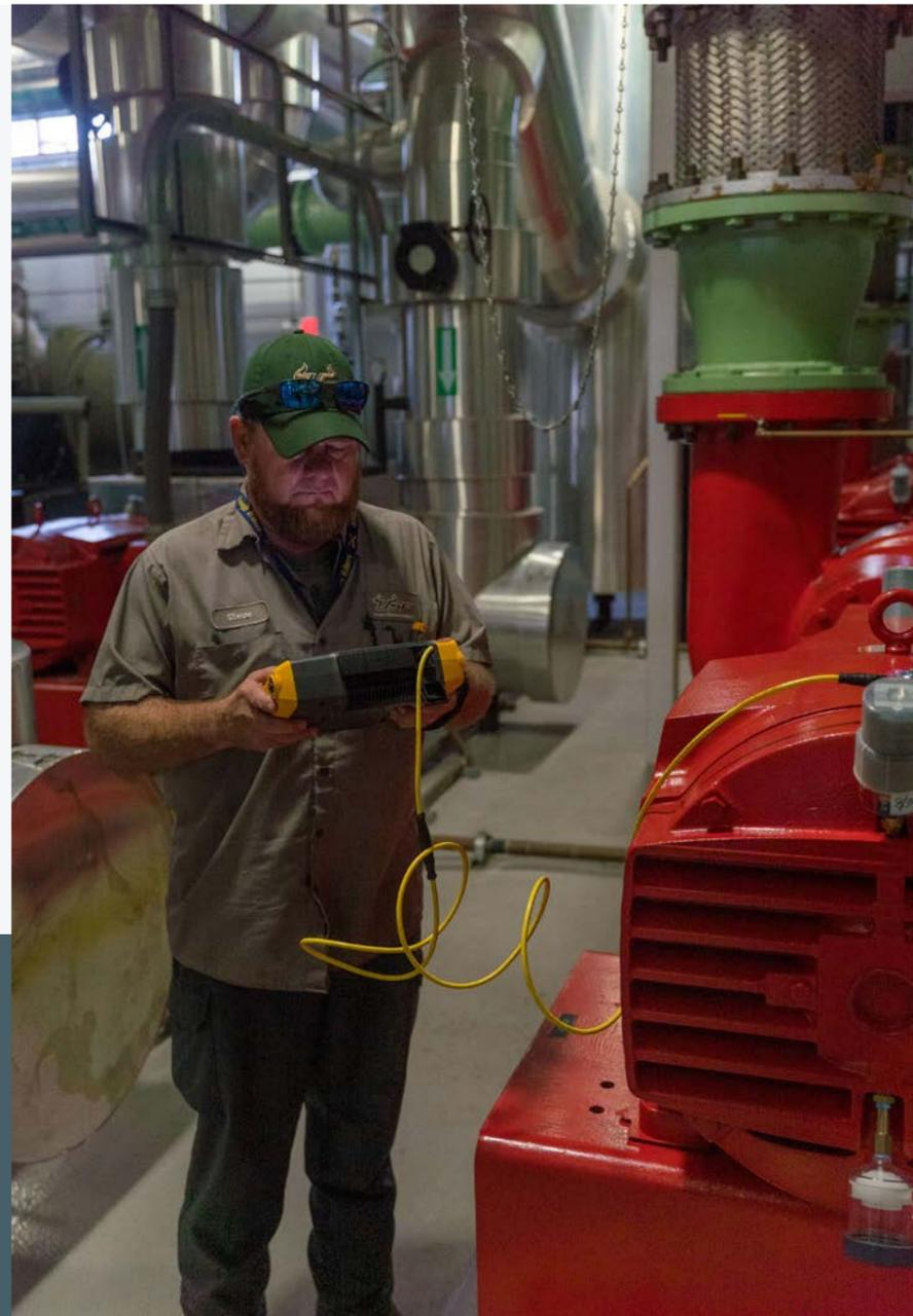
The Operations Department has implemented new predictive maintenance technologies like vibration analyzers and infrared cameras. These technologies are now part of the annual inspection process for centrifugal pumps and motors and have reduced maintenance costs, energy use, and labor costs in addition to increasing machine reliability by discovering anomalies before components fail.
