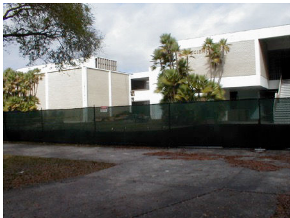
Before in preparation for demolition (Dec.27, 2014)
