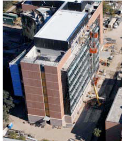
ISA Building facing the west side.
