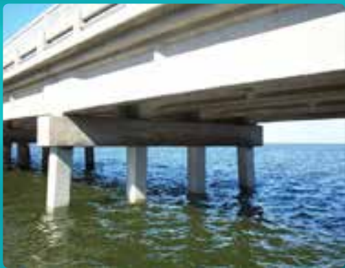
View of finished piles
