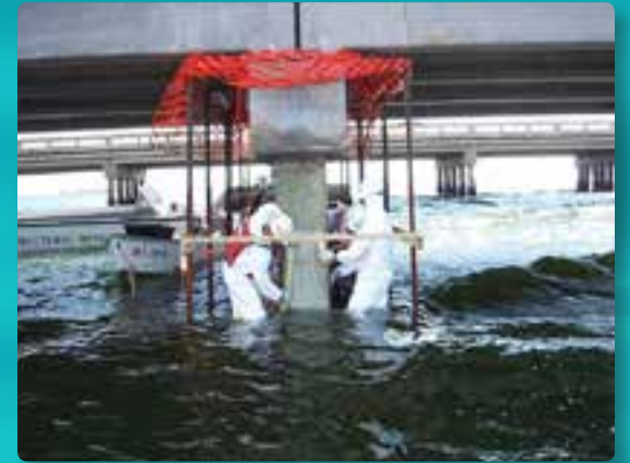
Set up for wrapping piles supporting Friendship Trail Bridge
