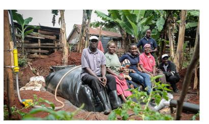
A biodigester in Kenya produces fertilizer and biogas for clean cooking in the home.
