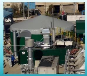
Built in 2015, this anaerobic digester runs on food waste only. It was designed to be very small because of its location in a crowded area. The Kishiwada plant exists to produce energy for the city of Osaka in Japan. Each year, 17 tons of food waste are converted to biogas and burned in a co-generation plant. The food waste comes from a waste processing facility that is nearby, so very little transportation is needed. This biodigester helps reduce the amount of waste produced by the city.
