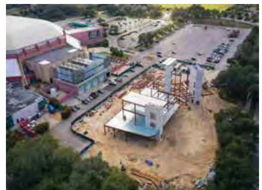
the new building progress through 21-22.
